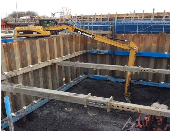
Properly designed excavation temporary works
