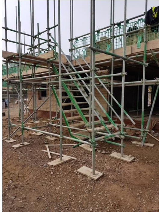
Very good scaffold access
