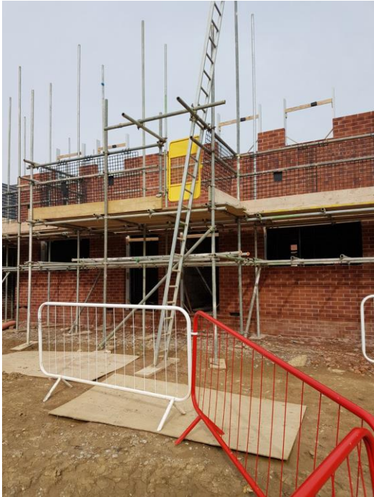
Good scaffold access
