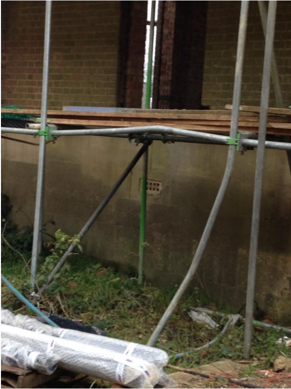
I'm sure scaffolding should be straight?
