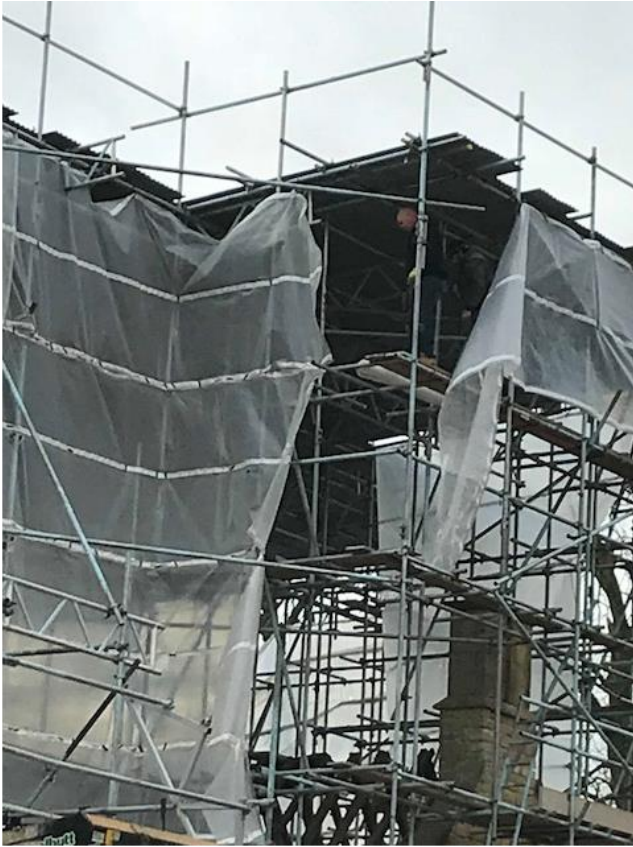
Spot the scaffolder? 😊
